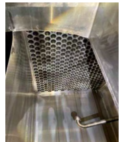
Bottom of Skim Milk Evaporator Tube Chest
